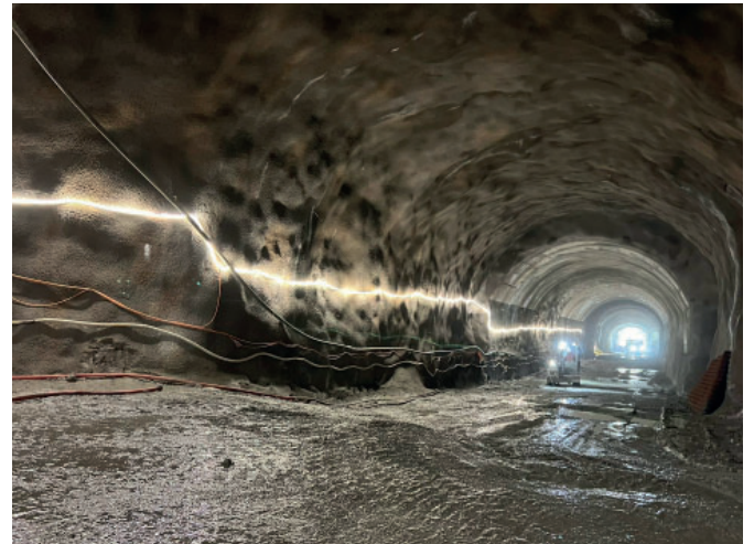
Implenia Switzerland, ARGE Gotthard
