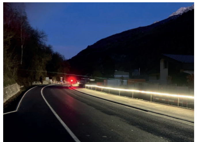
Construction site Bitsch VS
